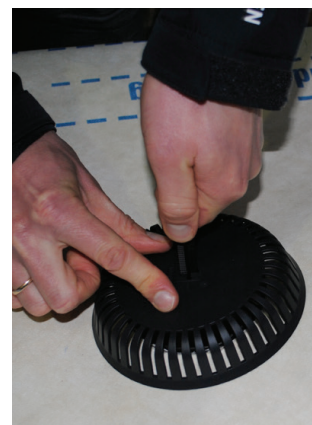
Overdelen presses ned mod undertaget
